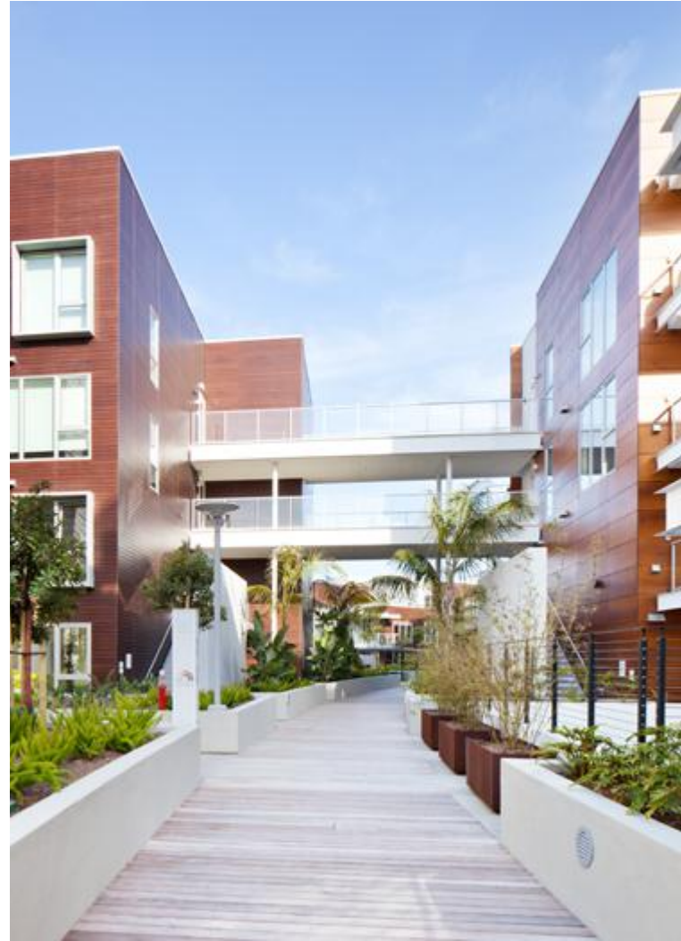
Product: NATURCLAD-W / Woods (from left to right): Pale, Onix, Rustik Residences in Pacific City, by MVE Architects (Huntington Beach, CA, USA)
