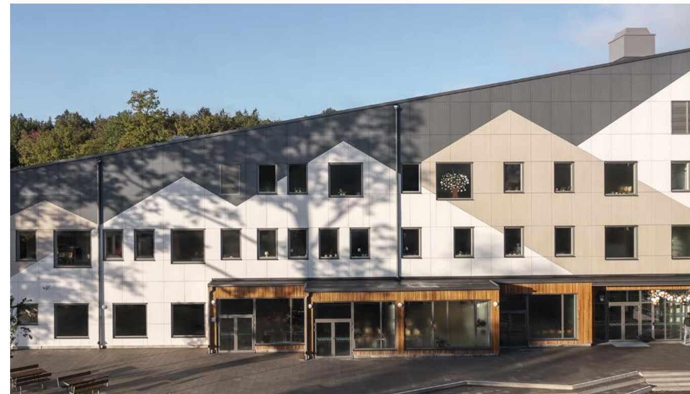
Långsjökolan Huddinge, Segeltorp, Sweden. Architect: Tyréns, Sweden and Arkitema Architects, Denmark. Photographer: Barabild Sverige AB, Stockholm, Sweden.
