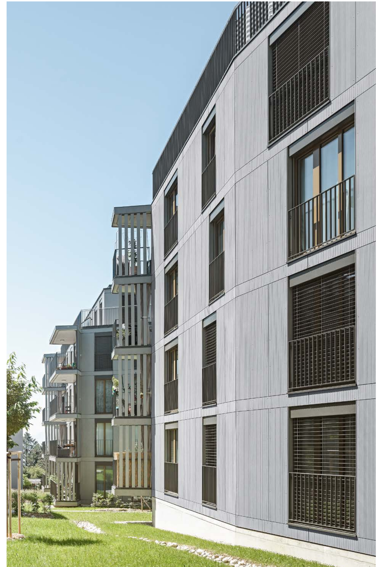
Fiches Nord, Lausanne, Switzerland. Architect: Züst Gübeli Gambetti Architektur und Städtebau AG, Zurich, Switzerland. Photographer: Roger Frei, Zurich, Switzerland.
