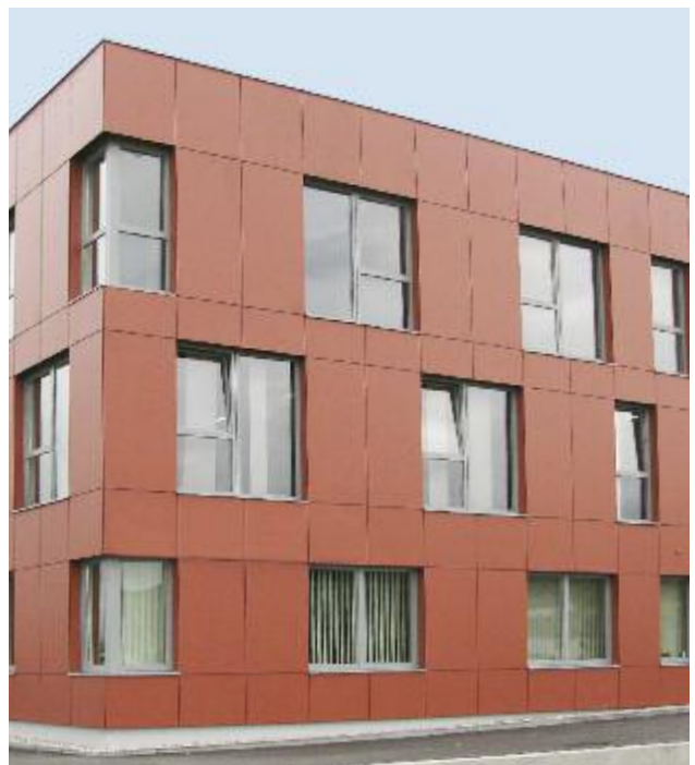
Facade cladding with NM surface
