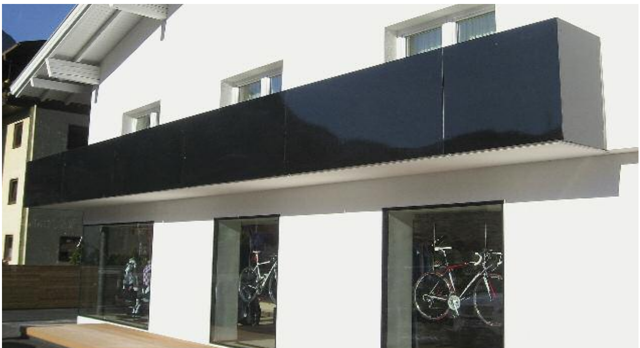
Balcony cladding/-design with NG surface
